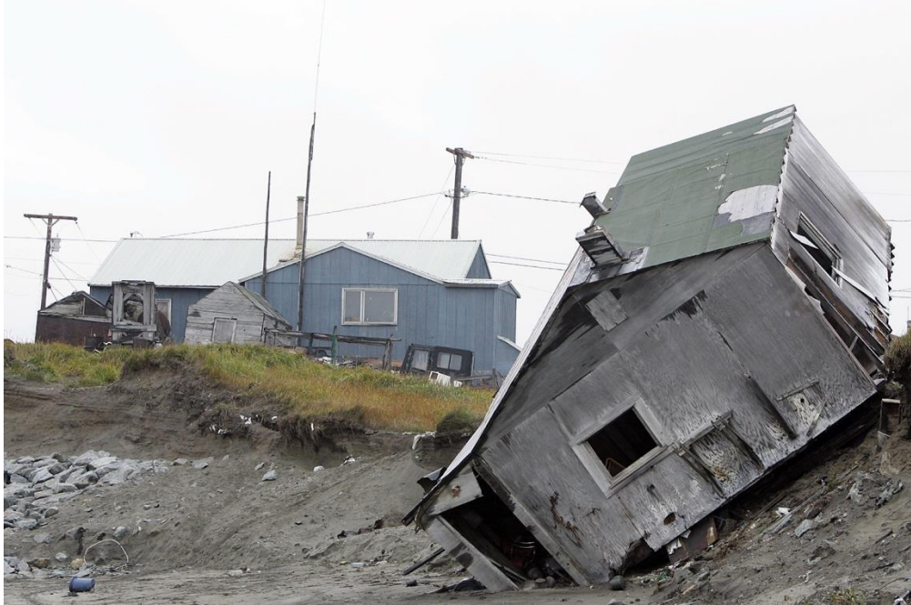
Image of a house that fell off the edge of the land in 2006 in the Shishmaref Community, Alaska. Photo provided by CNN.
